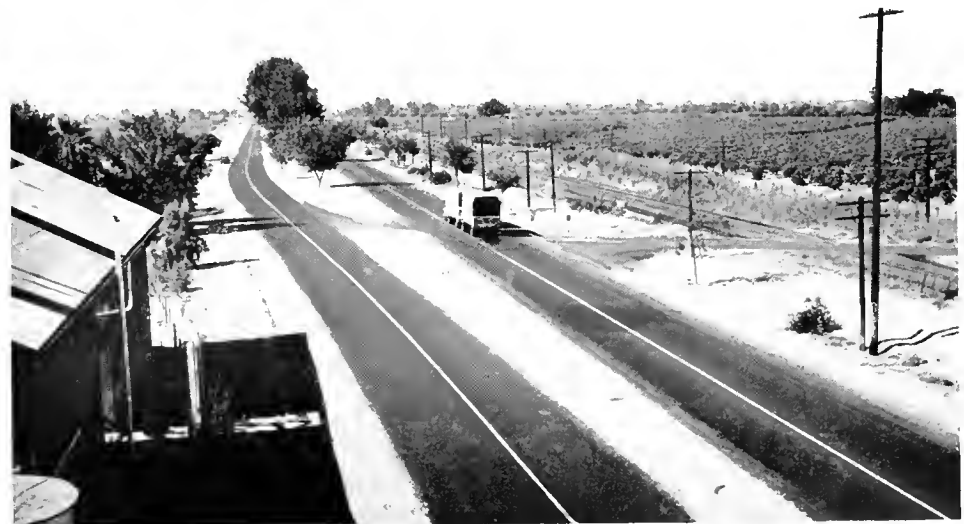
New divided road construction saves and utilizes on division strip trees that bordered roadside of old highway
